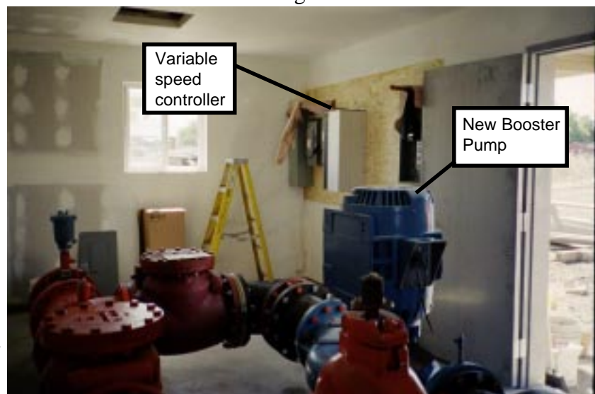
Figure 12. New booster pump during final installation.
