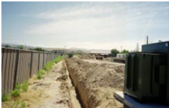
Figure 11. Underground electrical line extension to new booster pump house.
