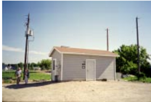
Figure 4. Well No. 4 pump.
