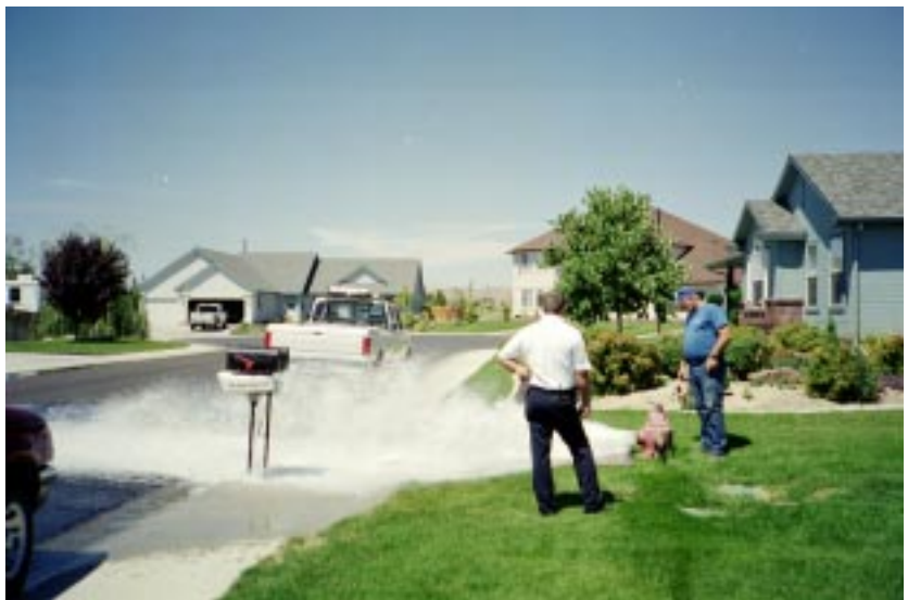
Figure 21. Fire flow test on July 27, 2000 at a hydrant located on N. Blacktail Place.
