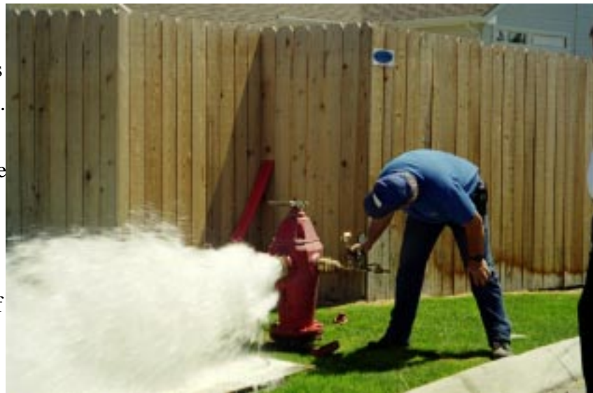
Figure 20. Norman Revels of Eagle Water Company check pressure during a fire flow test on July 27, 2000.
