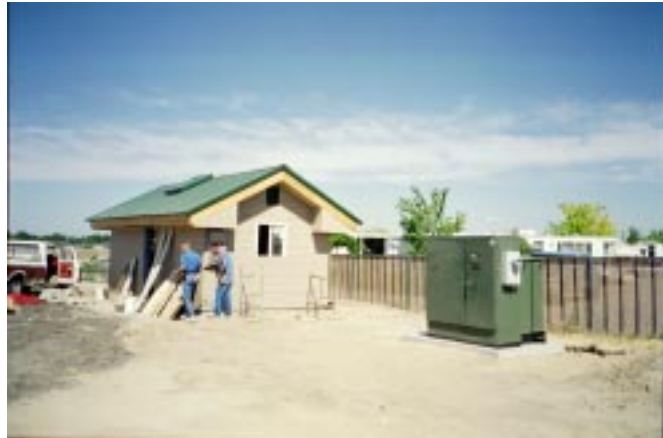
Figure 10. New booster pump house under construction.
